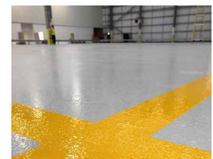
Safety line marking & cross-hatching
