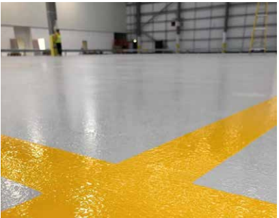
Safety line marking & cross-hatching
