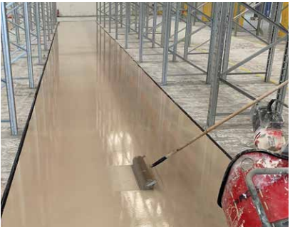
Cementitious levelling & wearing screeds
